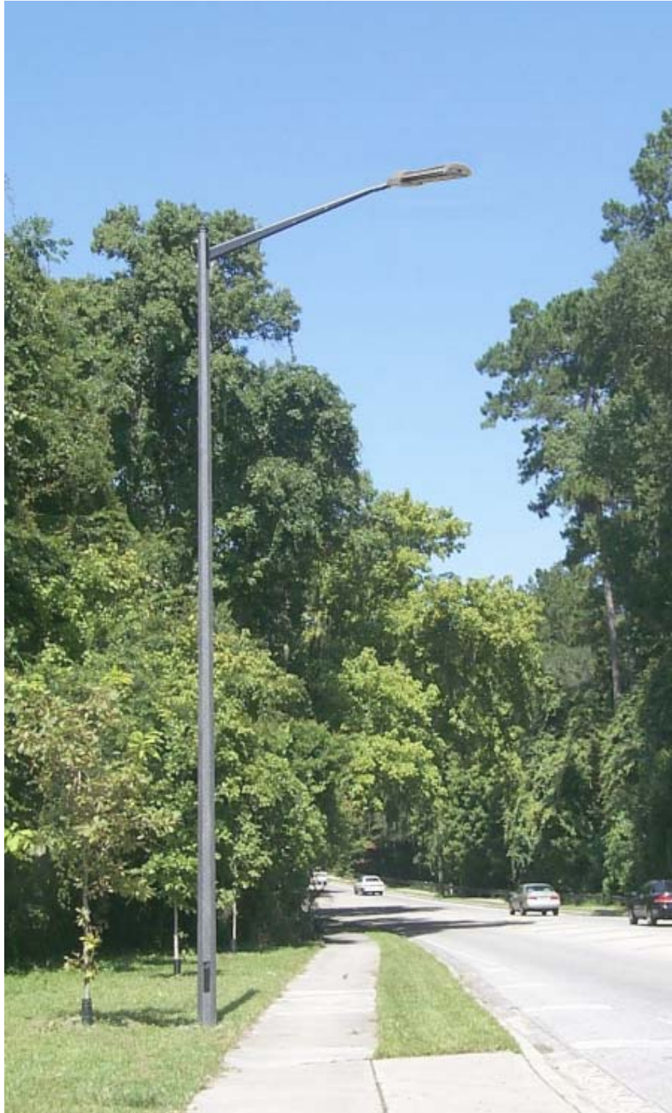
LED Roadway Cutoff - (Black) Light: (Light Type L42, L43, L44; Pole Type P14, P17)
